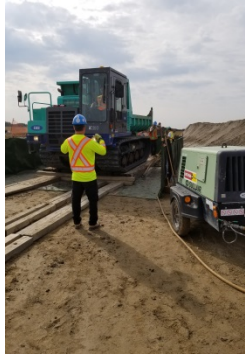
sept 11/18 Description & Location KP-822+125.6 Photo taken facing east Workers cleaning mud of the tracks
