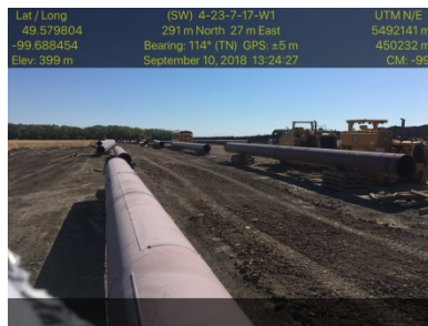
Sept 10/18 Description & Location: SSKP 908+000 Sections of pipe all End Prepped Ready to be welded For the Souris River bore Photo taken east
