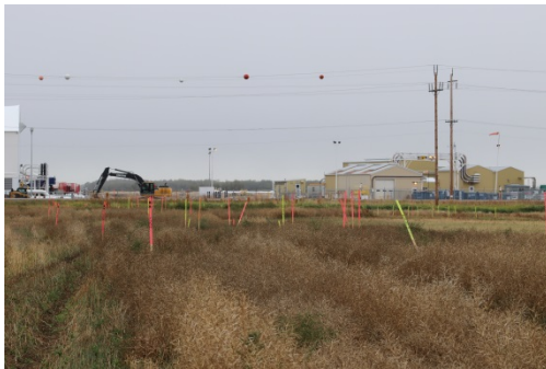
Sept 15/18 Description & Location: SSKP 865+000 West Souris Pump Station facing West Stakes indicating boundary and clipper line Farmers crops need to be removed
