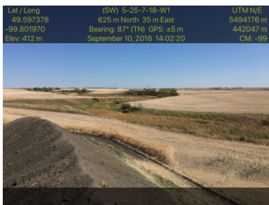
Sept 10/18 Description & Location: SSKP 899+760 Black Creek Water Course Work being done active all week Facing East
