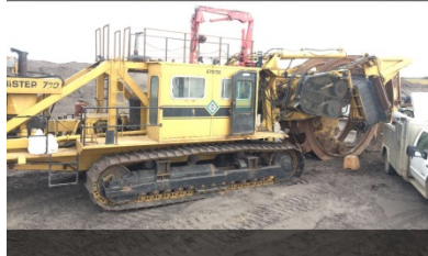
Sept 13/18 Description & Location: SSKP 813+100 Ditcher has arrived as of yesterday Side boom holding bore head in sling Mechanic is doing maintenance getting it ready 54 foot digging wheel Will start ditching crew on Sept.24th
