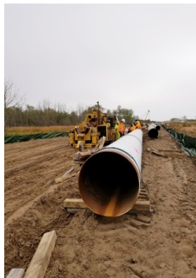
Sept 14/18 Description & Location KP-819+239 Photo taken facing west workers getting pipe ready for the bending machine
