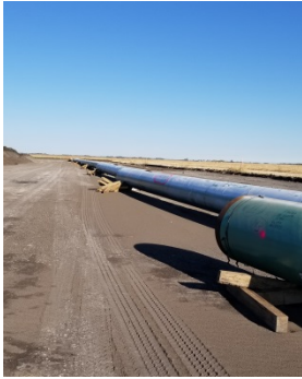
Sept 10/18 KP_813+200.0 Photo taken facing south. Unloading pipe
