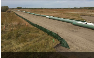
Sept 13/18 Semi-Permanent Marsh Class 4 MB-1039 Stringing crew has pipe ready for End Prep Facing NW
