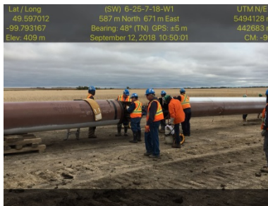
Sept 12/18 Description & Location: SSKP 899+760 Getting ready to line up pipe and start the root weld, the pipe was previously pre-heated before this process photo North
