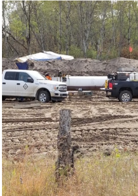
Sept 12/18 Description & Location KP-819+500 Photo taken facing north. Worker's welding the pipe at SF # 12
