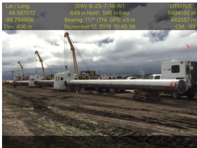
Sept 12/18 Description & Location: SSKP 899+760 Poor Boy crew cleaning and checking bevels making sure good, pre-heating. The automatic welders doing a Root, Hotpass and Cap, photo taken SE
