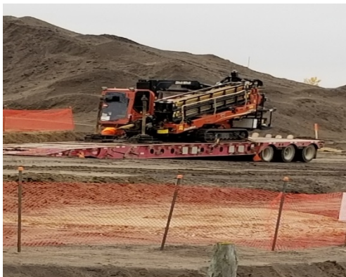
Sept 15/18 Description & Location KP- 838-132.8 Photo facing north Equipment operators waiting to get machines washed
