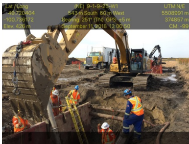
Sept 11/18 Description & Location: SSKP 828+222 Hydro-vac sucking water up Excavator removing clay and water Drilling crew changing out reamer In Wetlands facing South West
