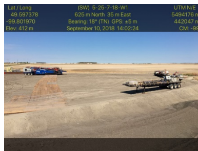
Sept 10/18 Description & Location: SSKP 899+760 HDD pad for Black Creek Entry hole for bore will start here
