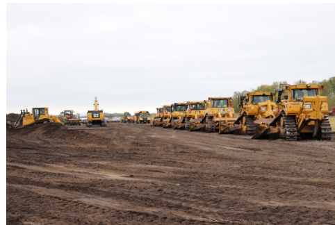
Sept 15/18 Description & Location: SSKP 836+600 Cleaning section 200 m west Dozers lined up waiting to be cleaned Dozer to left pushing topsoil Photo facing west
