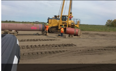
Sept 13/18 Description & Location: SSKP 826+450 Welders helpers prepping bore for welding
