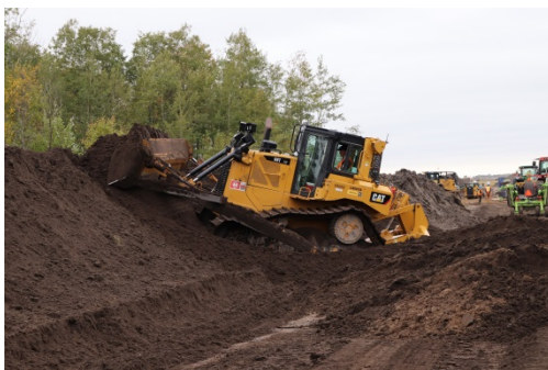
Sept 15/18 Description & Location: SSKP 836 + 700 Dozer pushing and piling topsoil Photo facing west
