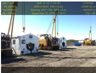
Sept 10/18 Description & Location: SSKP 899+950 3 automatic welders 18 sections to weld for Black Creek bore Photo taken East
