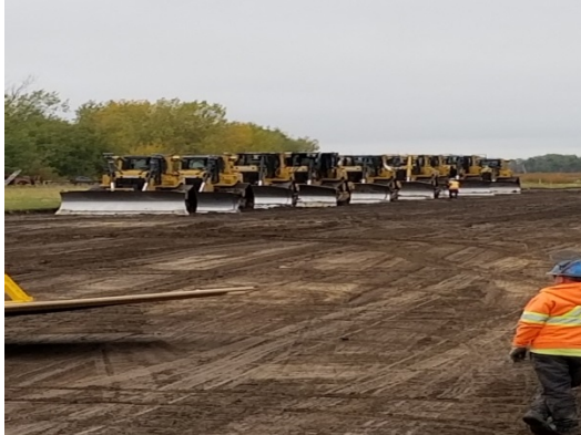
Sept 15/18 Description & Location KP- 838-132.8 Equipment operators waiting to get machines washed
